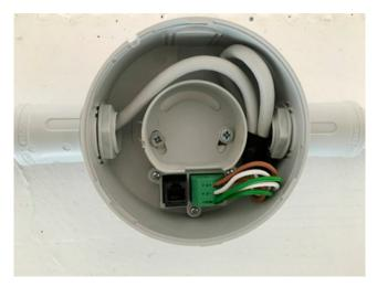
Place the wire around the inner part of the base to avoid damage of the isolation of the cable.
